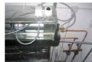
Office Fancoils Installation
