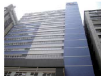
Yoochoo Tower 800 ton Water Cooled HVAC System Design+Build
