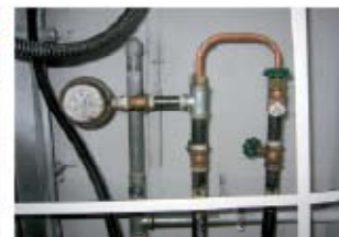
Chiller Pipes Pressure Test
