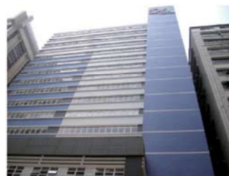
Yooahoo Tower 800 ton Water Cooled HVAC System Design+Build
