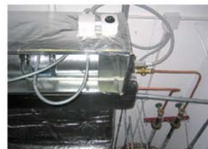
Office Fancoils Installation
