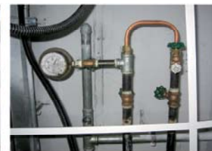
Chiller Pipes Pressure Test
